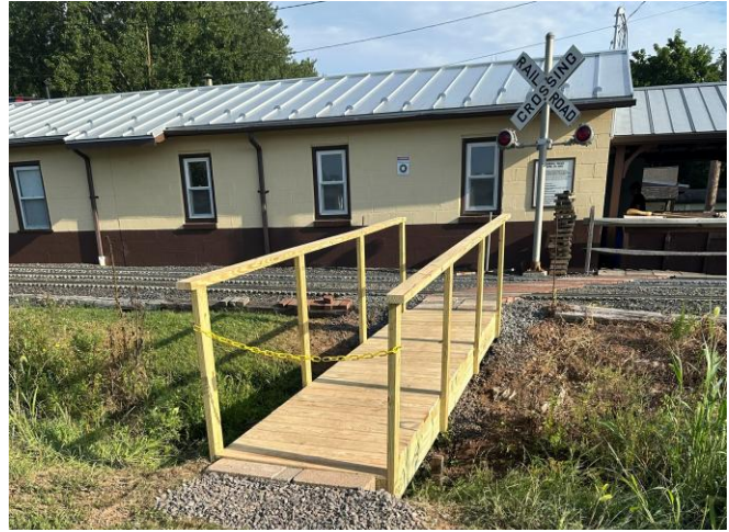
New Bridge after installation.
