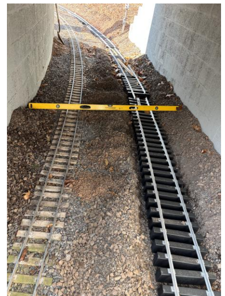
This shows the tight alignment in the tunnel on 36" centerlines.
