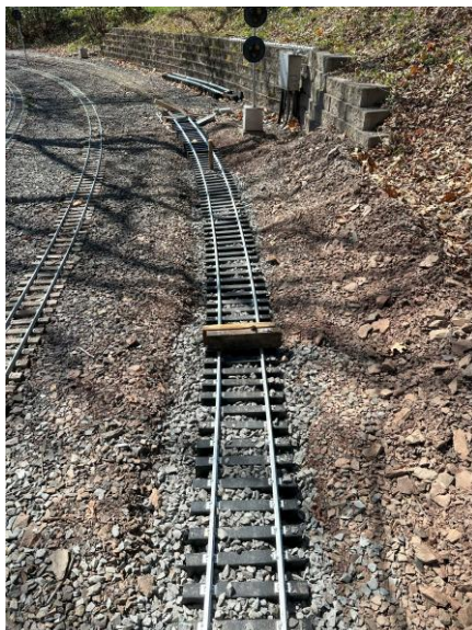
This shows where the grade will climb a little to meet the elevation at the Yard Turnout.
