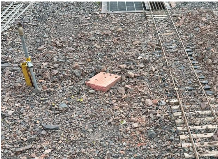
The new Yard Air Tap right next to the Water Tap and the hole is back filled ready for Tamping the Yard Track.
