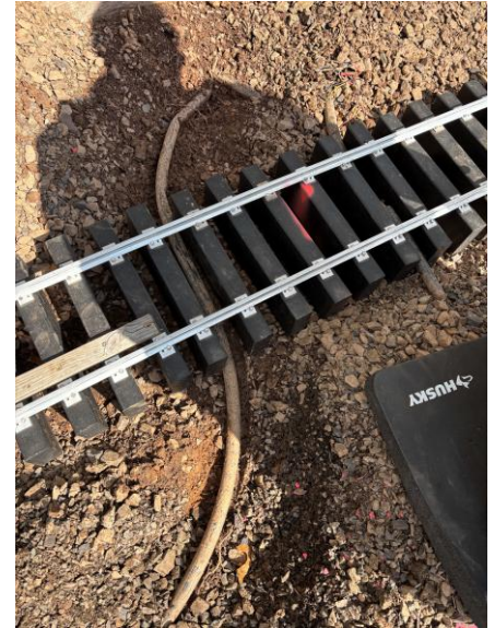
We had to be careful with the existing signal system conduits.
