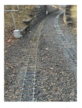
Another view of the progress on the 7.25" Main east of the Station. Some of the water-soaked ties have been replaced. The next area to be worked after the Station exit is inside the Tunnel and then on the Mercer Bridge.
