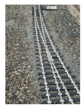
This is the 3<sup>rd</sup> Turnout rebuilt in place. This one is on the 4.75" Main near to Bldg. 8. The before picture was in the last Gazette.
