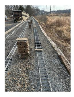
Remove & Replace Ties Project continues as some of the worst Ties along the South property line are replaced. Also, some of Railroad Ties were replaced. They were all installed in 1999 and endured the hot Sun and a few floods.
