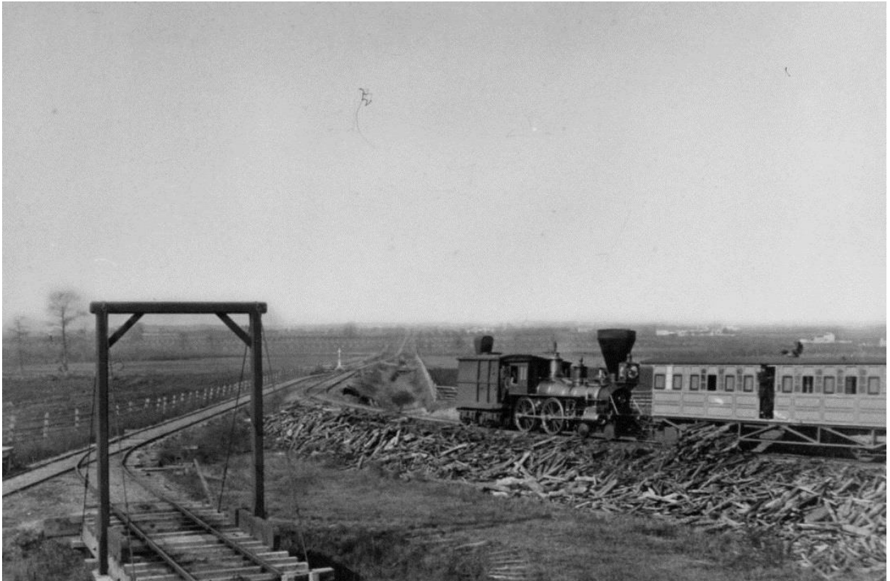
Circa 1863 photo of the Princeton Branch at Princeton Junction Station (looking west towards Princeton). Note the primitive turntable for turning the locomotive. The station is to the train's right.
