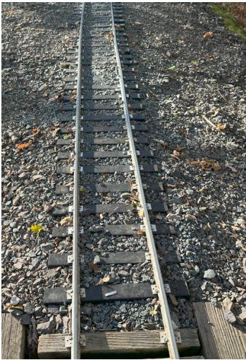
South going from Mercer Bridge
