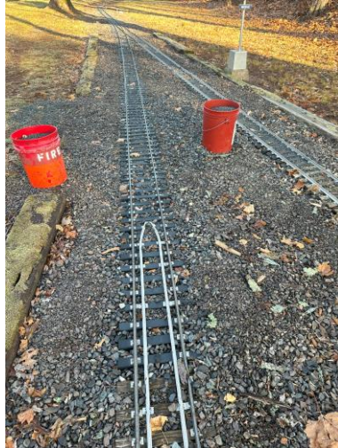
Looking towards the Tunnel
