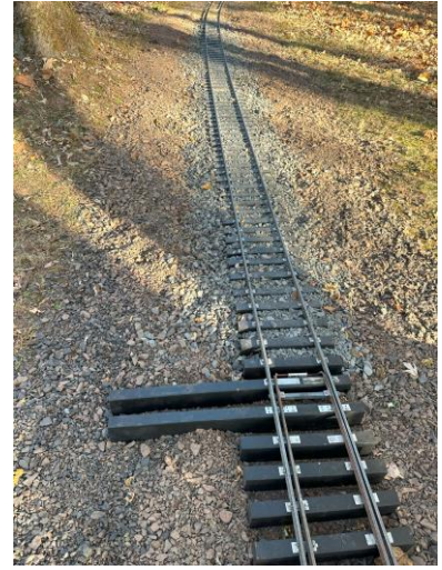
The North end just short of the Tunnel.
