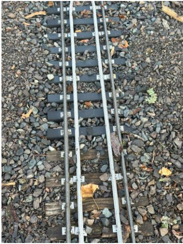
Current end of the Project just short of the Twin Bridges.
