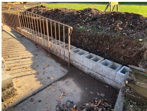
BLOCK BEING REINSTALLED
