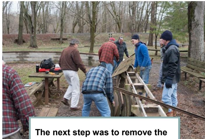
**The next step was to remove the old deteriorating roadbed.**
