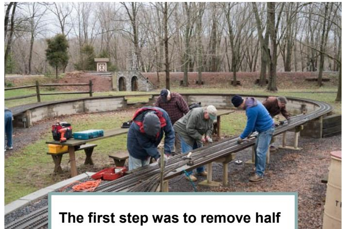
**The first step was to remove half the existing track and turnouts.**
