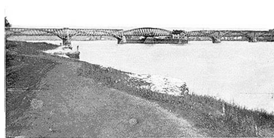
Top: Lithograph of the bridge on fire fifteen days after its completion. Below: The first bridge as rebuilt after the collision and fire.
