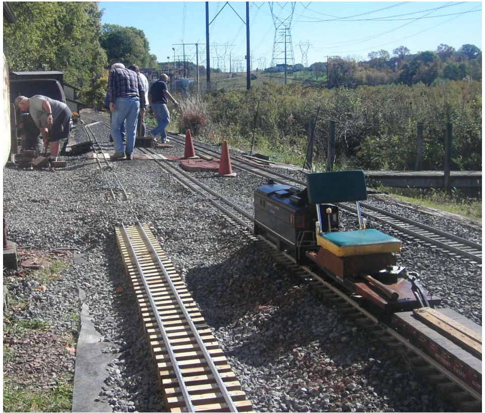
Ballast is applied to the new siding as the work train stands by with the compressor.
